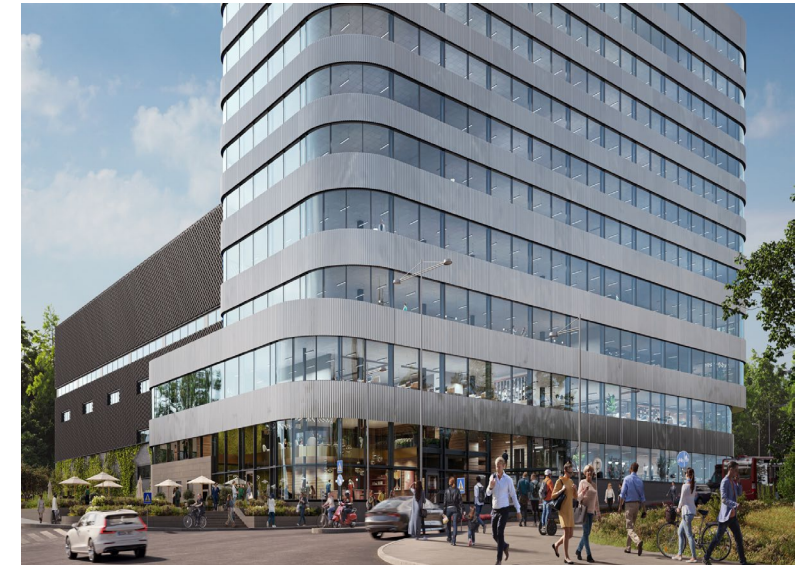
Alfa Laval, (Separatorn 1) Flemingsberg
